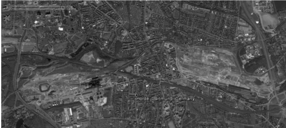
Fig. 4 Iron and steel works area Hoerde-Dortmund, situation 2006 (Google maps)
