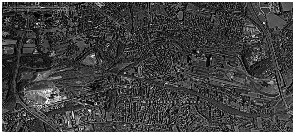
Fig. 3 Iron and steel works area Hoerde-Dortmund, situation 2002 (Google maps)
